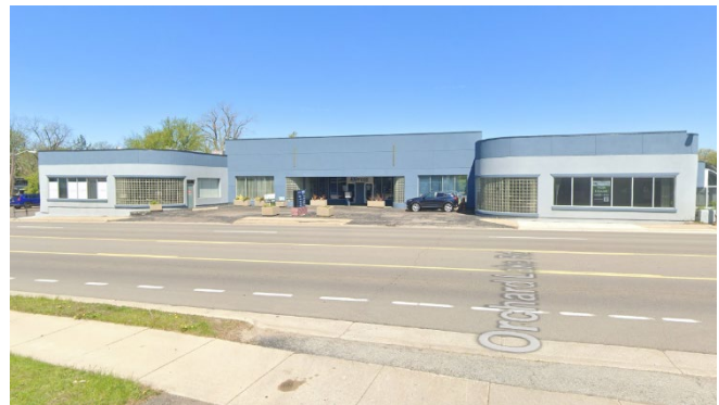
Existing site conditions as shown on Google Street View in May 2025.
